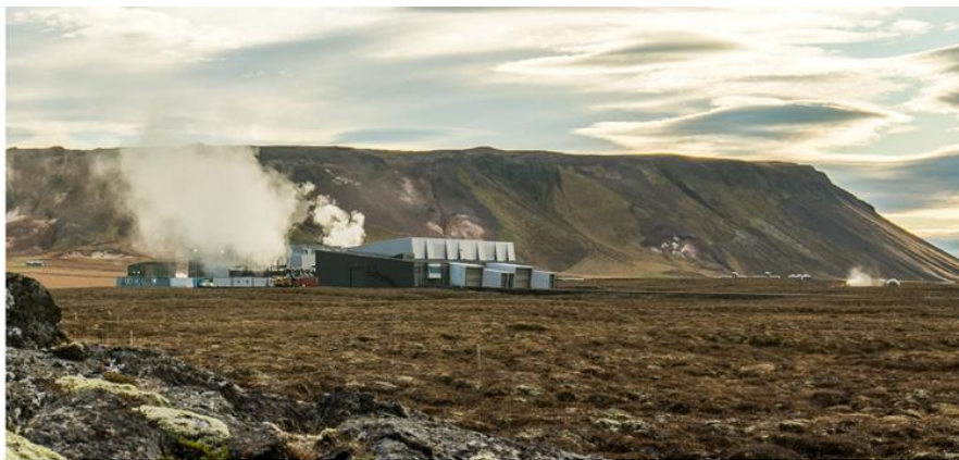
Figure 6: Theistareykir power plant. Photo: Mannvit.
