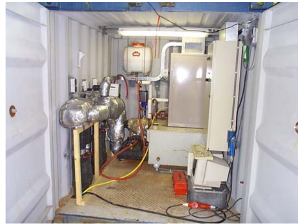
Figure 1: Mobile TRT test rig with heat pump
