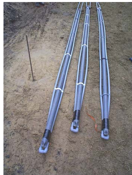
Figure 8: Single-U vertical heat exchanger
