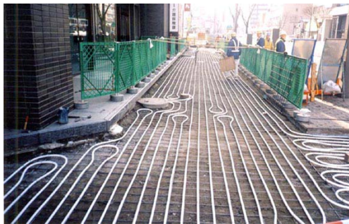
Figure 15: Installation of heating pipes (East Unit).
