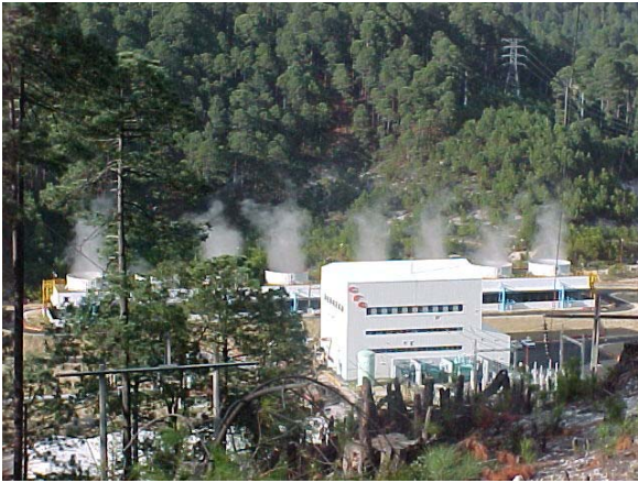
Figure 7: Condensing unit of 50 MW (U-7)
