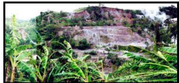
Figure 6: This is the quarry in Upper Mahiao in LGPF where the upper load was reduced and the slope face benching to prevent further slippage.
