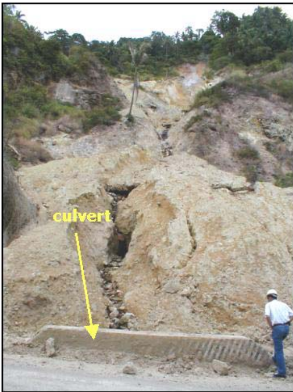
Figure 4: Photo shows the slide materials coming from the Mag-aso thermal ground in the Southern Negros geothermal field being diverted to a large culvert below the road.
