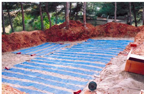
Figure 4: Picture of an earth-coupled geothermal heat pump installation in Thessaloniki.
