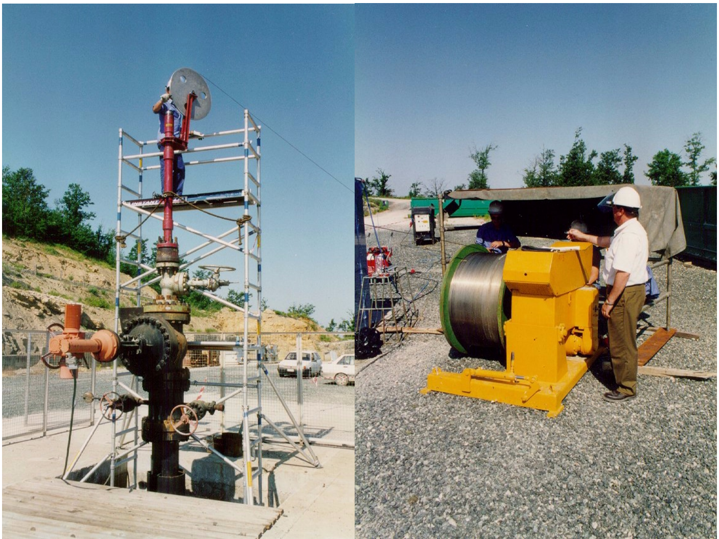
Fig. 3: Injection line and pump station
