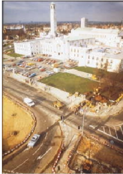
Figure 2. The heating mains being laid across one of the busiest junctions in the City Centre.
