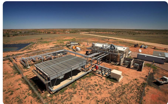
Figure 3: Habanero Pilot Project (HPP) 1MW Plant (source GDY Internal)
