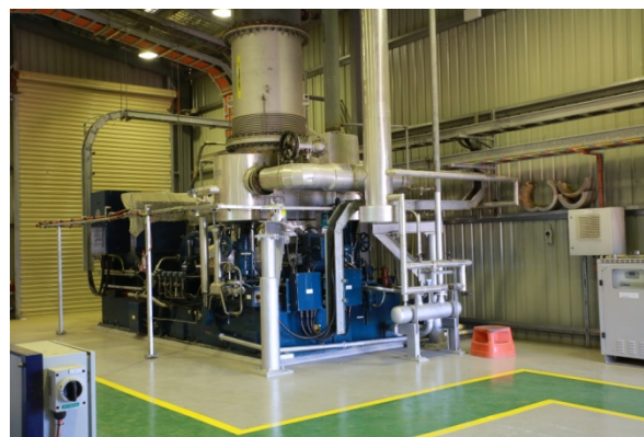
Figure 5: The steam turbine of the 1MW Plant (source GDY Internal)
