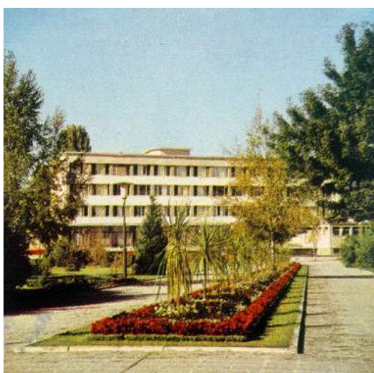
Fig.4. A sanatorium, heated with geothermal energy
