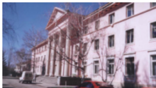
Fig.6. A sanatorium heated with geothermal energy
