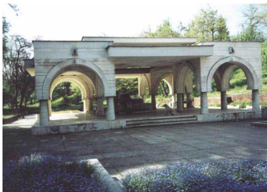
Fig.13 Thermal water fountain (Hisarja town)
