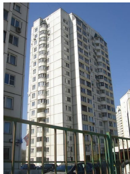
Figure 3: Moscow, Anokhina Str., 62. An example of a building in Moscow with supply of heated water, using heat pumps.
