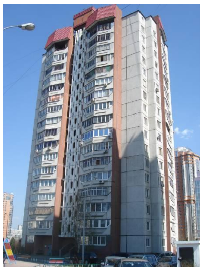
Figure 2: Moscow, Anokhina Str.,50. A building of pilot heat-pump installation. An example of a building in Moscow with supply of heated water, using heat pumps.
