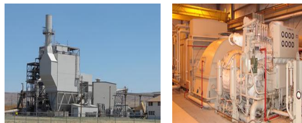
Figure 4 and 5: Honey Lake power plant (Source: Greenleaf LLC 2012)
