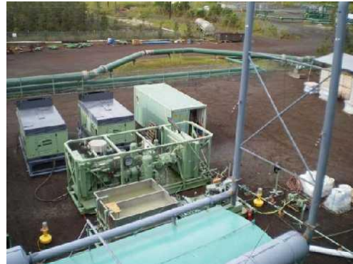
Figure 2: Part of the equipment installed by Air Drilling Associates
