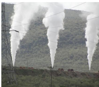
Figure 2: OW 44 series discharging. The wells discharge a combined capacity of 20MW
