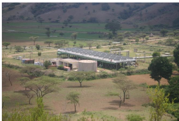
Figure 1 The Aluto Pilot Geothermal Power Plant
