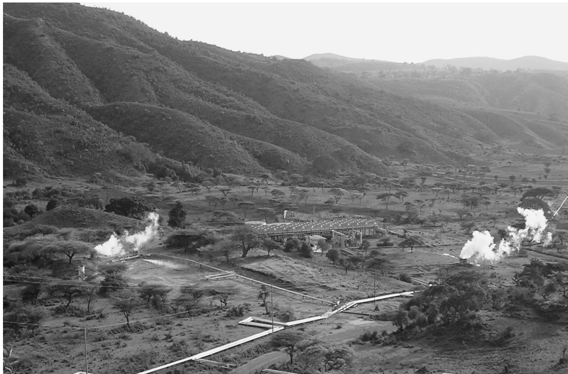
Figure 3. Aluto Langano Gpp in Operation
