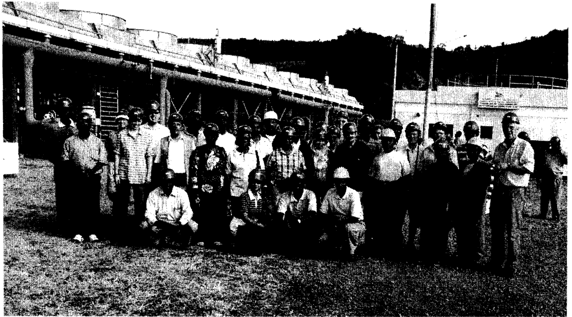
Pre-Conference field participants at the Aluto-Langano Geothermal Pilot power plant, Ethiopia. (November 25, 2006)
