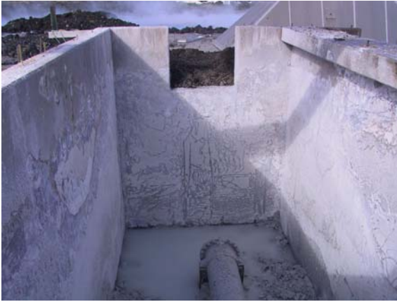
Figure 10: Silencer after cleaning. Inlet pipe can be seen on the bottom.
