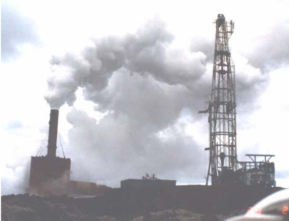
Figure 5: Workover showing rig and silencer.
