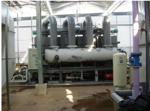
**Figure 4: 45 RTon commercial four-bed adsorption chiller, US Patent US6490875, Singapore Patent 82589**
