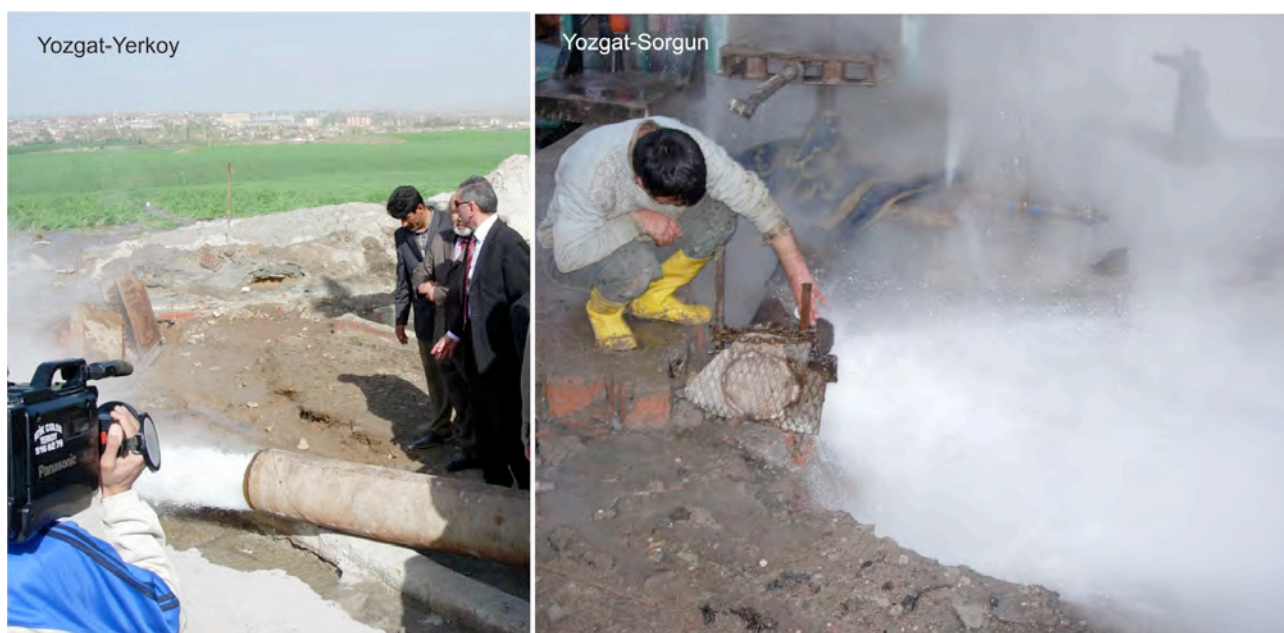
Figure 4. Drilled wells for geothermal heating applications in Yozgat.
